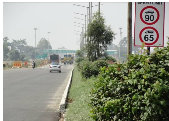
Fig 4: Wrong Signage near Toll Barrier (RD 145.000 Km)
