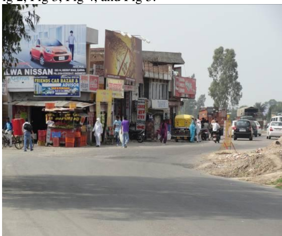
Fig 2: Lack of Proper Diverging Lane (RD 143.400 Km)
