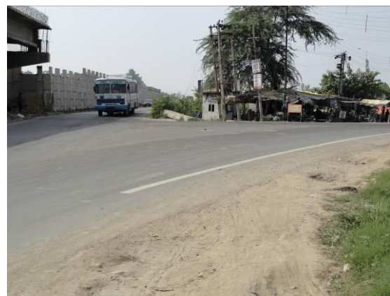
Fig 5 Road Side Development on Y- Junction (RD 129.030 Km)
