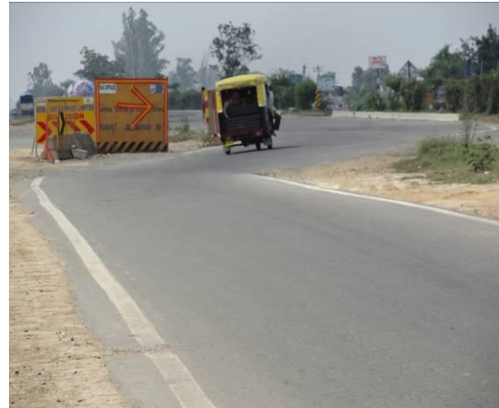
Fig 3: Sharp Diversion (RD 140.000 Km)
